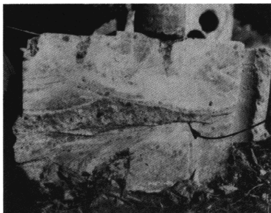
VOIDS BEHIND REINFORCING STEEL
