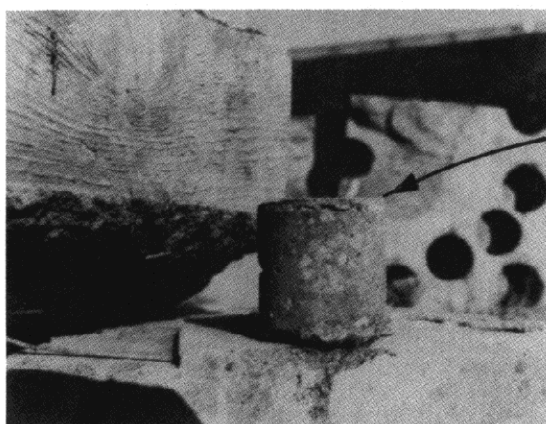
DELAMINATED FLASH COAT ON FINISHED SURFACE OF SHOTCRETE
