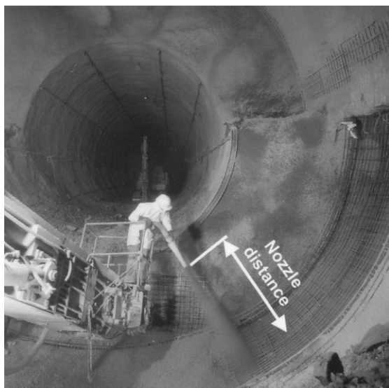
Figure 86: The distance of nozzle to substrate influences rebound and compaction.
