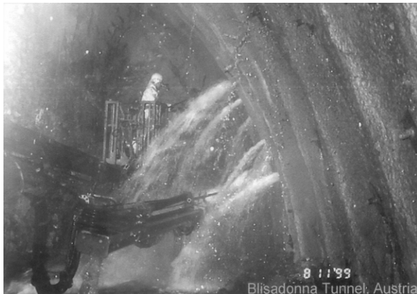
Figure 83: Water ingress controlled through pre-installed pipes before application of sprayed concrete
