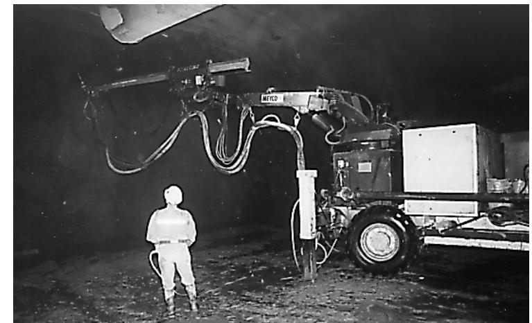
Figure 27: Modern sprayed concrete: Robotic spraying with advanced admixtures and steel fibres
