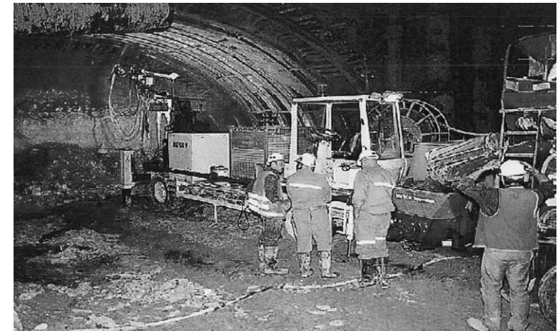
Figure 75: Robotic spraying provides superior sprayed concrete quality.
