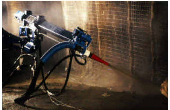
Figure 4: Robotic manipulator for safe, high output and quality wet-mix sprayed concrete application
