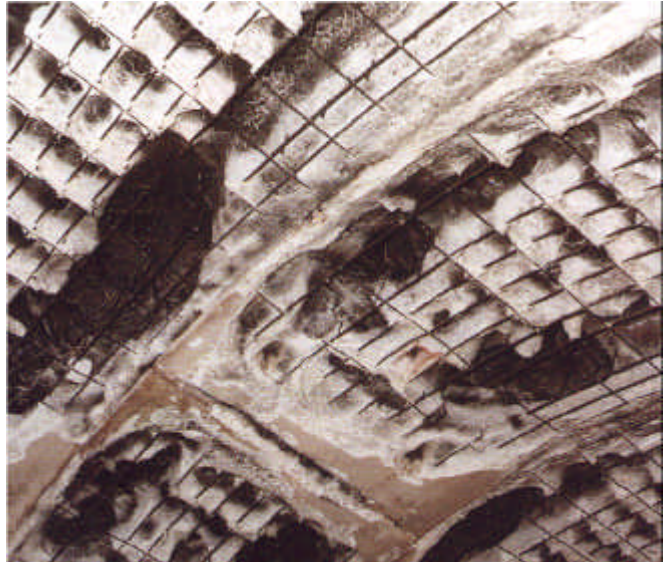
Figure 14: Channel Tunnel fire damage
