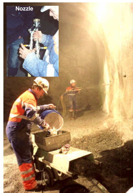
Figure 12: Using a simple screw pump, two men can apply sprayable membrane up to 50m 2 per hour
