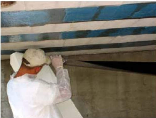
c) Application of CFRP Laminates
