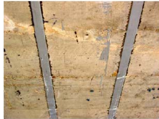
d) Application Completed
