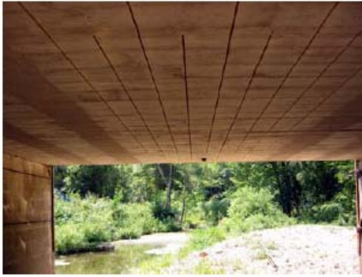
a) Grooves Prepared as per Design Geometry
