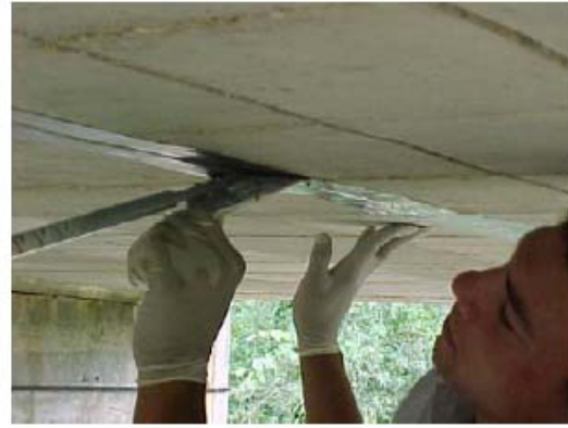
b) Inserting Epoxy Paste into the Groove
