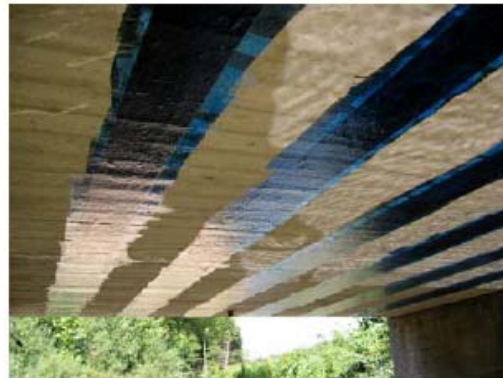
d) Application Completed
