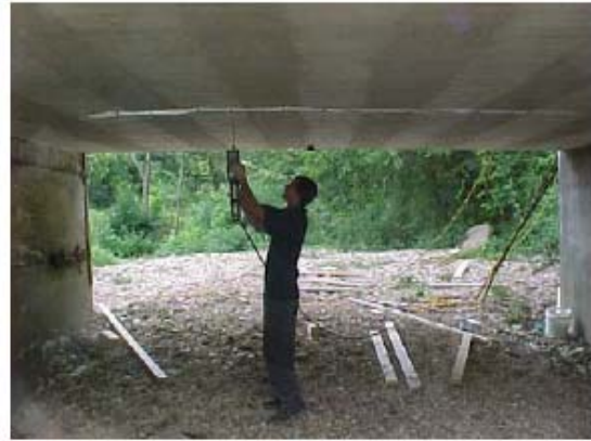
b) Crack Injection under the Bridge
