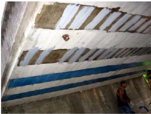
a) Surface Preparation with Primer and Putty
