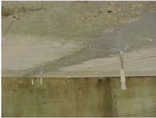
a) Crack Sealed Previous to Injection
