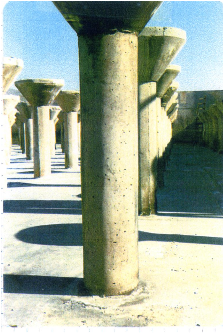
General view, after the earthquake.
