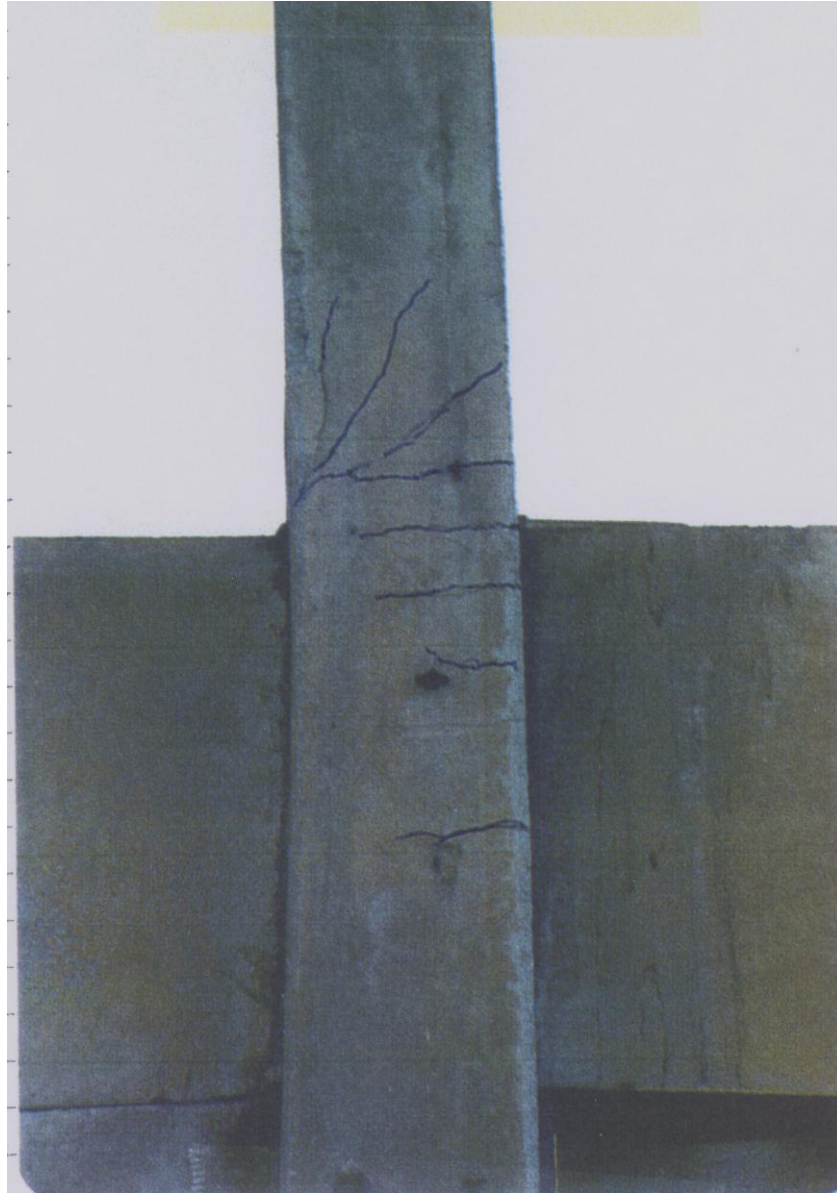
Damaged captive column (interaction with the CP's).
