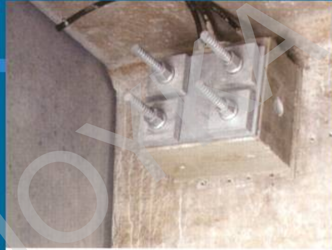
Finished anchor block
