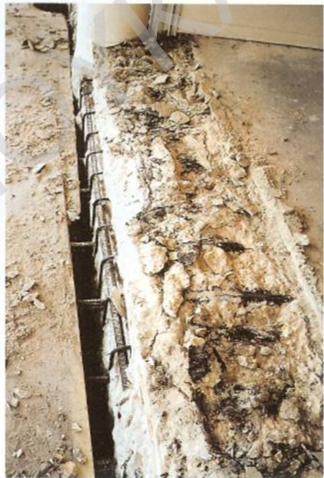
View of same area before repair
