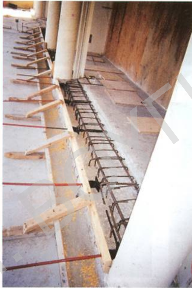
Correct repair of post-tensioned slab edge/beam
