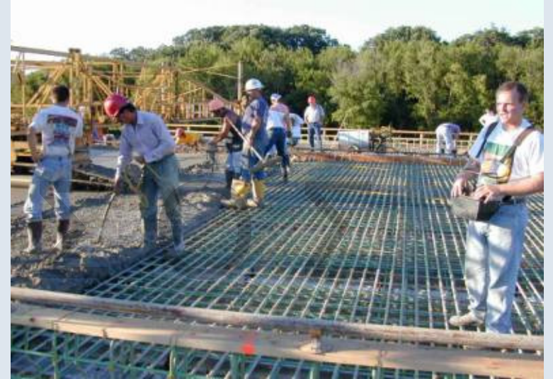
53 rd AVENUE BRIDGE
